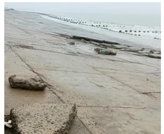
Fig.9: Slab collapse due to faulty construction of the concrete embankment in Mousuni island, Kusumtala block. Source: Photographed by author. Date:25 th August,2023.
