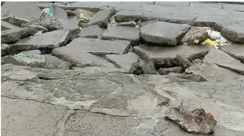
Fig.9: Slab collapse due to faulty construction of the concrete embankment in Mousuni island, Kusumtala block. Source: Photographed by author. Date:25 th August,2023.
