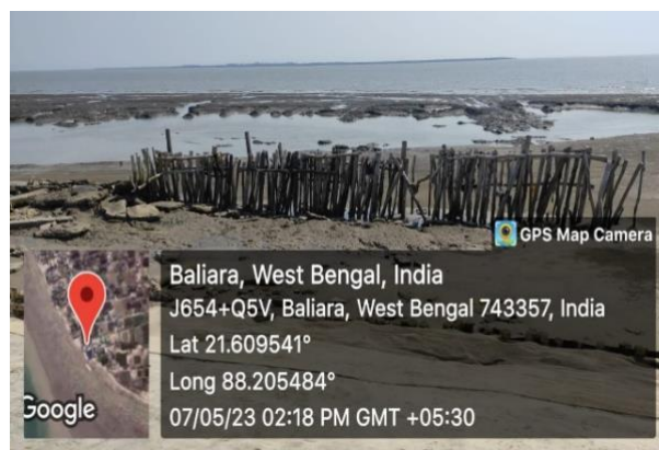
Fig.6: Wooden log embankment Source: Picture captured by author. Date: 7 th May 2023
